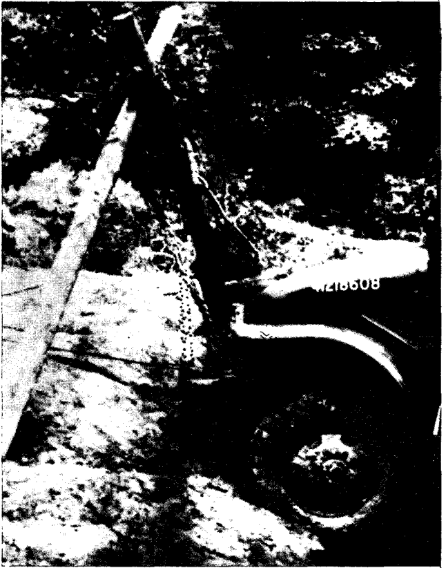
Figure 44. Recovering a nosed truck with an A-frame.
